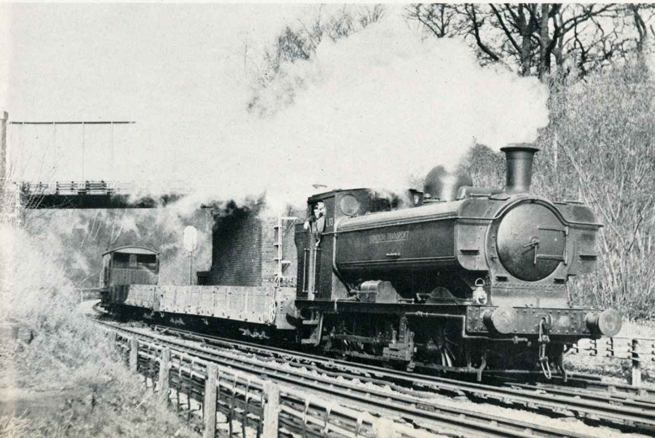
105 A former GW 0-6-0PT, London Transport No. L93, curves round from the Watford branch to join the Metropolitan main line near Moor Park with a ballast train.
